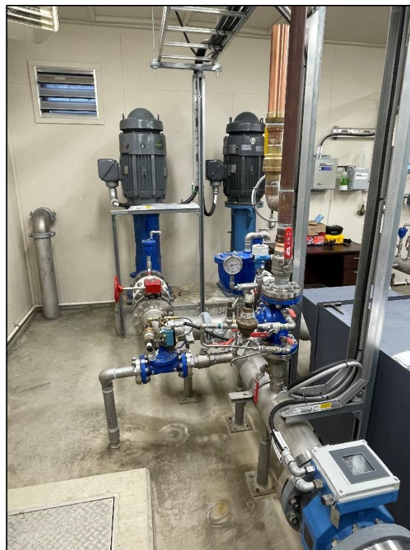
Treatment Station Booster Pumps
