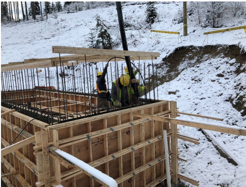
Figure 1: Construction of Wet Well at Booster Station
