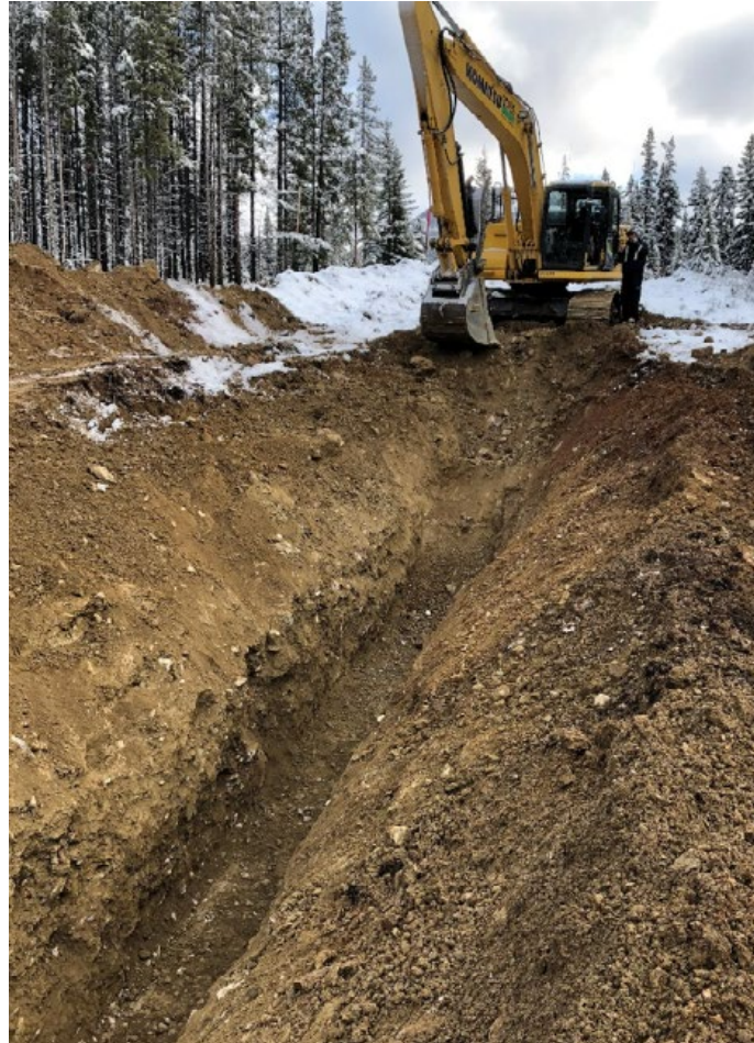
Figure 2: Excavation for Waterline from Booster Station to Reservoir
